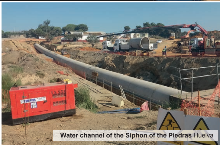
Installation concrete pressure pipe with steel cylinder
