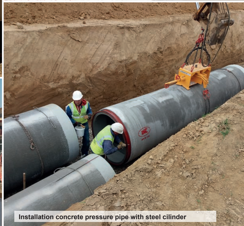
Fittings of concrete pipe with steel cylinder
