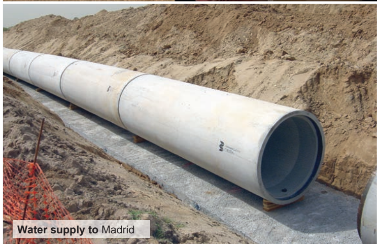
Concrete pipe with double elastic joint
