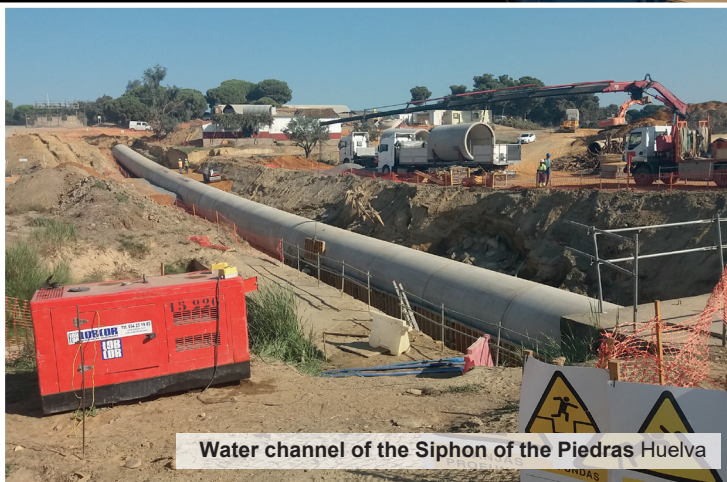
Installation concrete pressure pipe with steel cylinder
