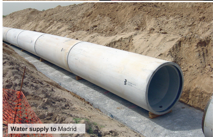
Concrete pipe with double elastic joint
