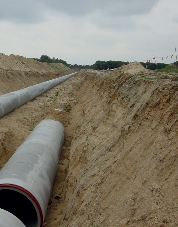
Transport of concrete presure pipe with steel cilinder
