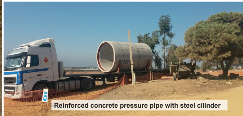
Transport of concrete presure pipe with steel cilinder
